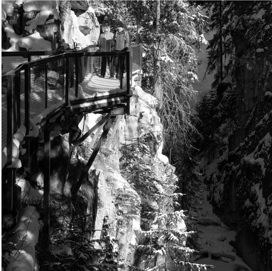
In Johnston Canyon, a snowpacked trail follows the creek, partly along suspended metal catwalks.
